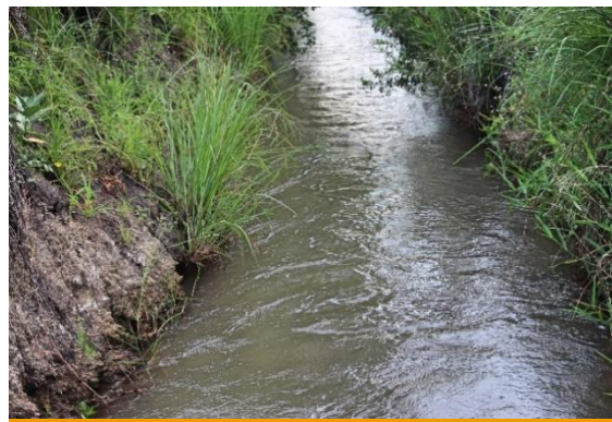
Figure 3.5. Conveyance canals at the lower end
