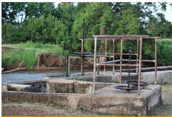
Figure 3.4. Tulo Kongwa weir 1
