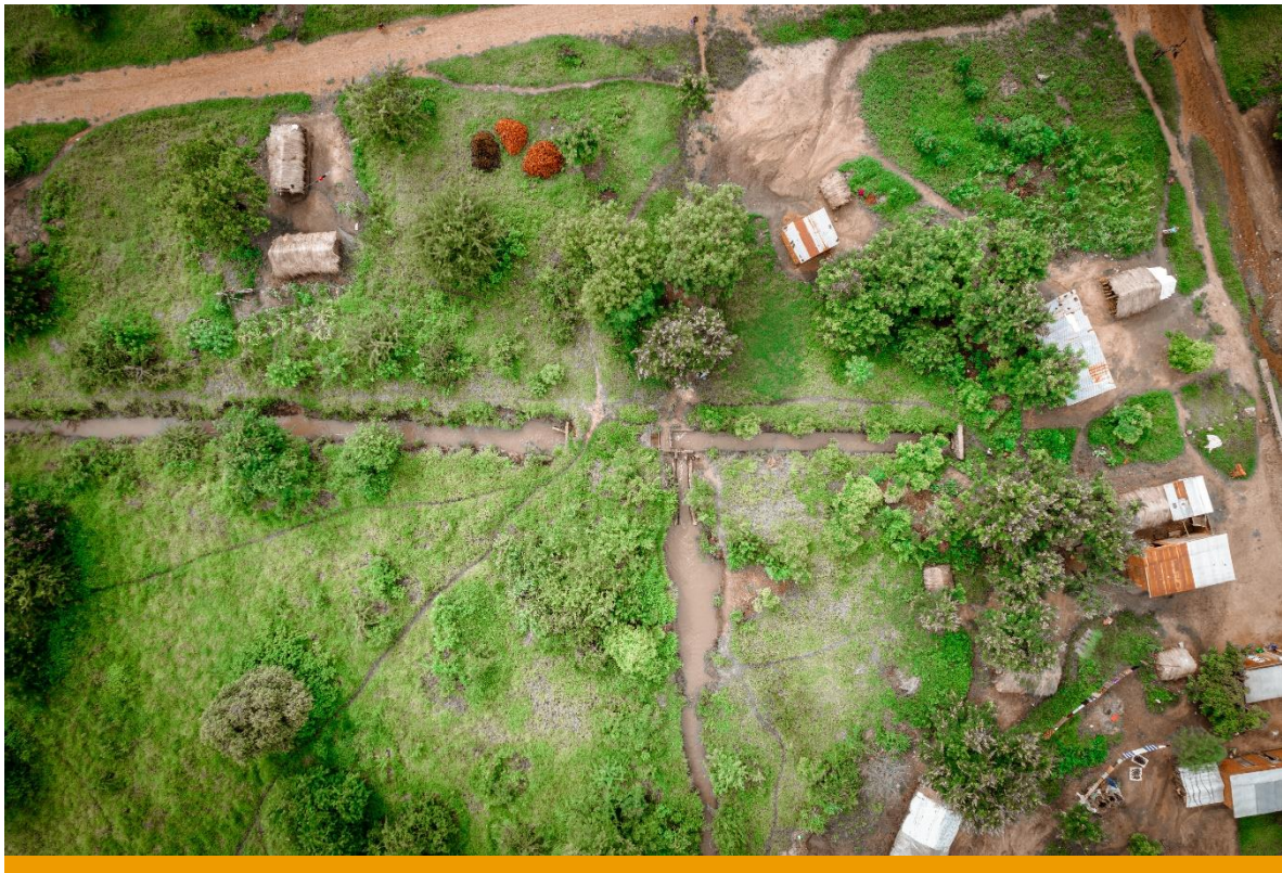
An aerial view of a different section of the Tulo Kongwa irrigation scheme. This section is also unlined.
