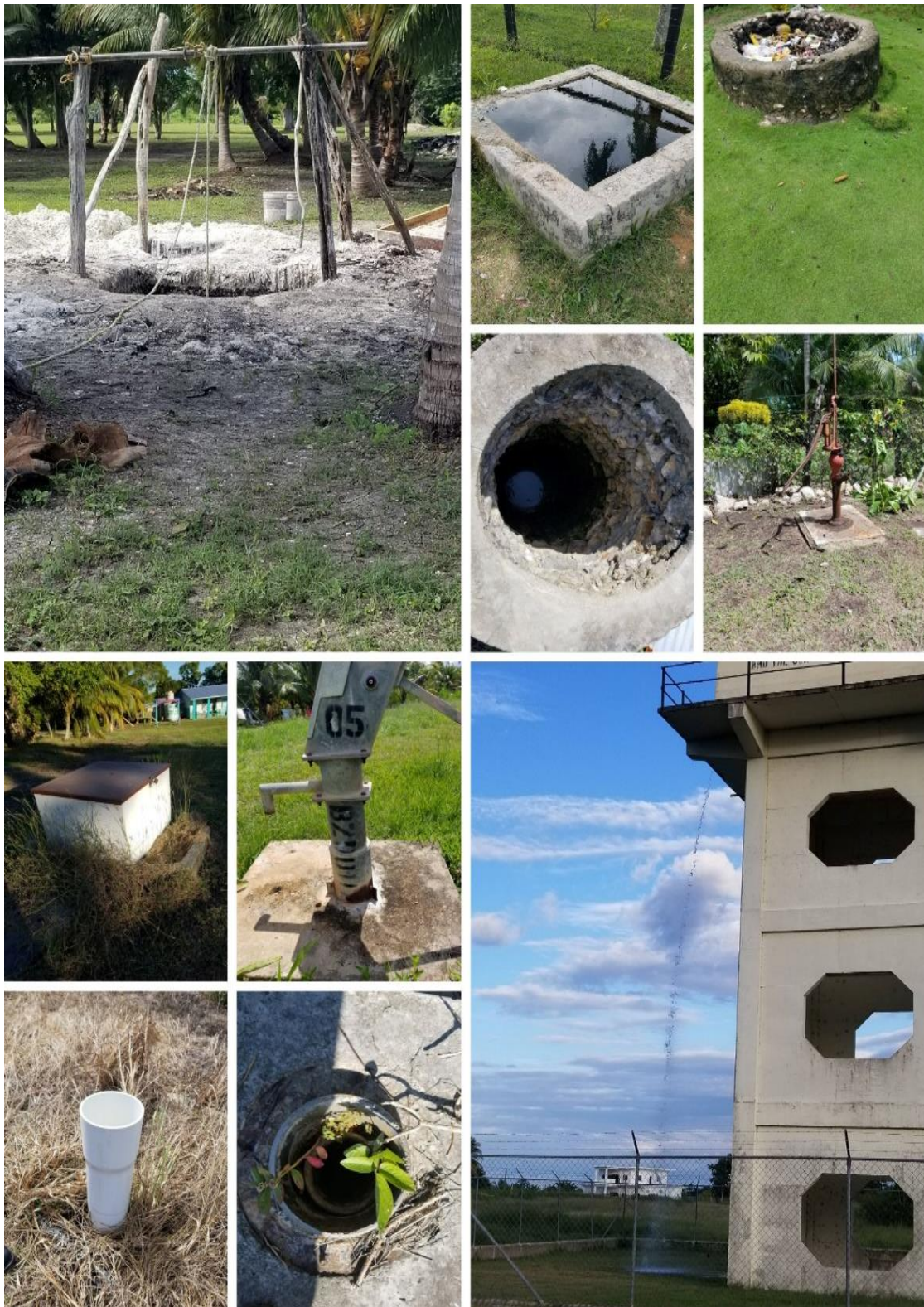
Figure 1: Some of the wells and pumps in northern Belize that were visited during the on-site data collection.
