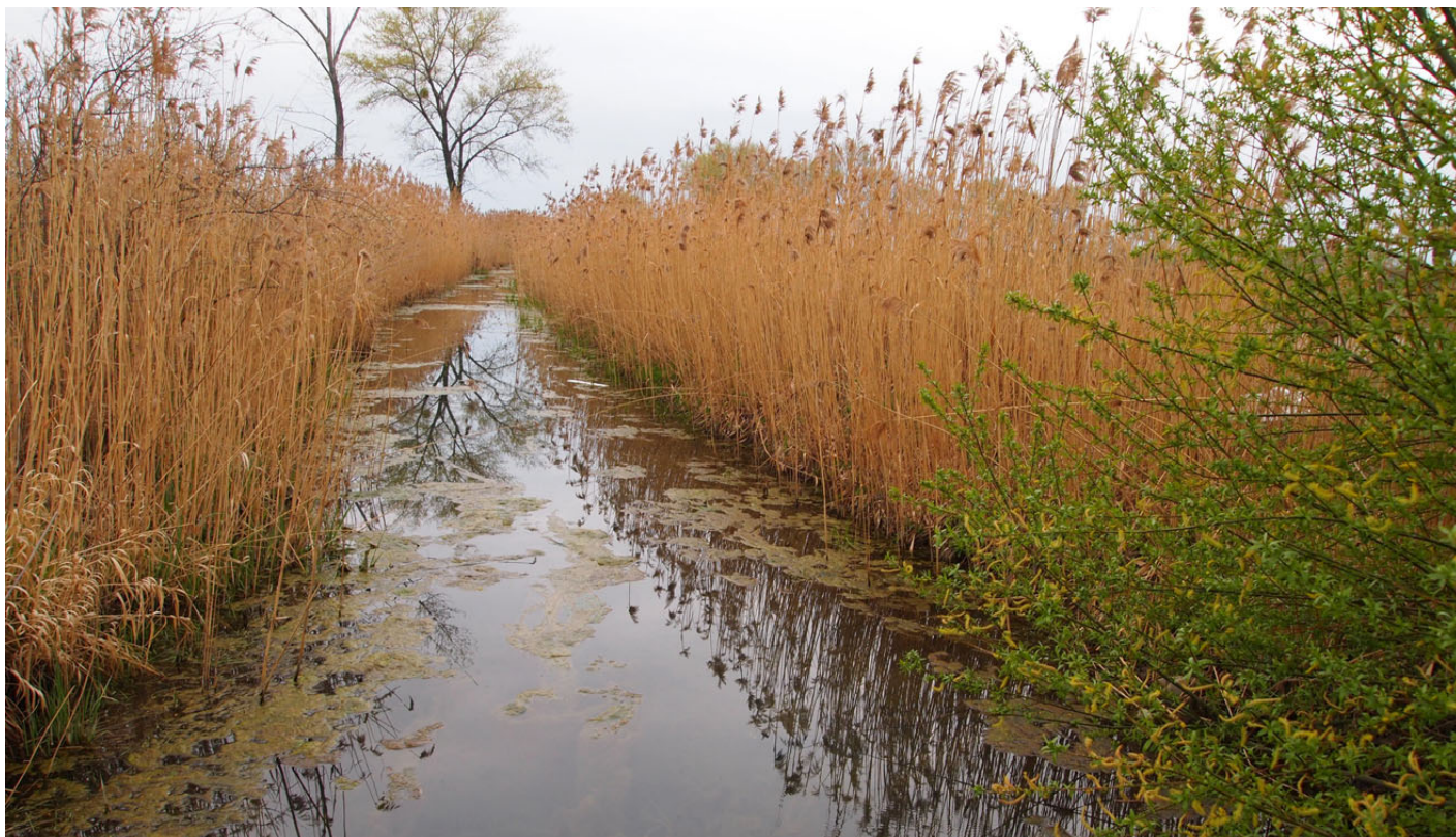
Reed beds are used as a method of removing pollutants from waste water
