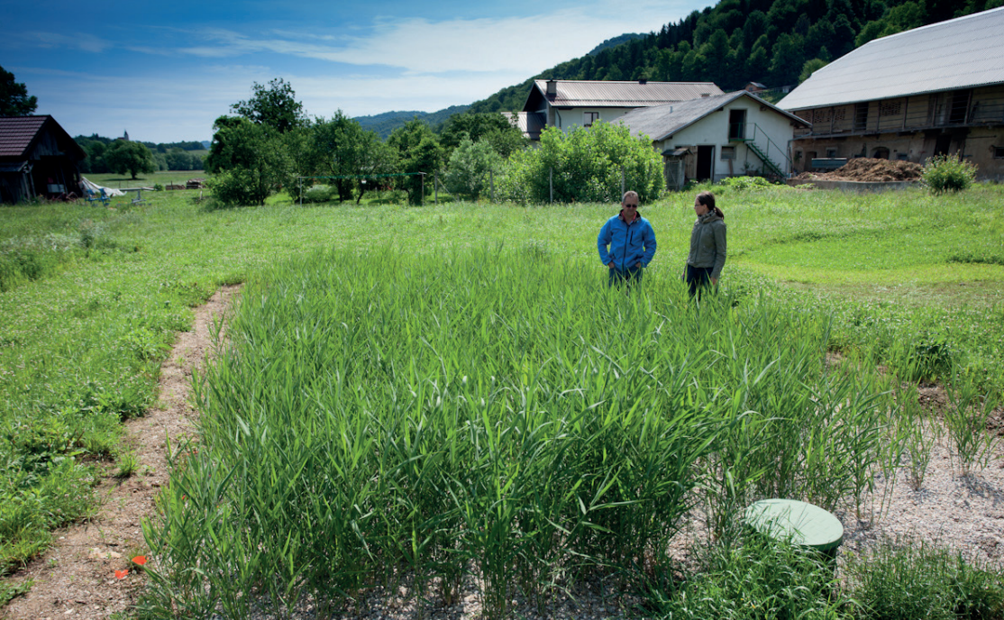
Picture: Constructed wetland for treatment of wastewater from a single household. (Photo: Iztok Ameršek)
