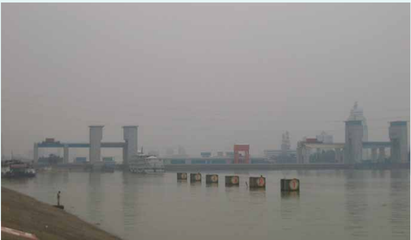
Gezhouba Dam on the Yangtze River, and the upstream approach to the ship locks Credit: Vmenkov via Wikimedia Commons
