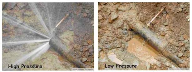
Figure 7. Burst water main at high and low pressure (photos: Ronnie McKenzie, WRP, Ltd.)
