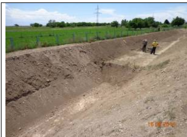
Construction of the pool system for second waste water treatment
