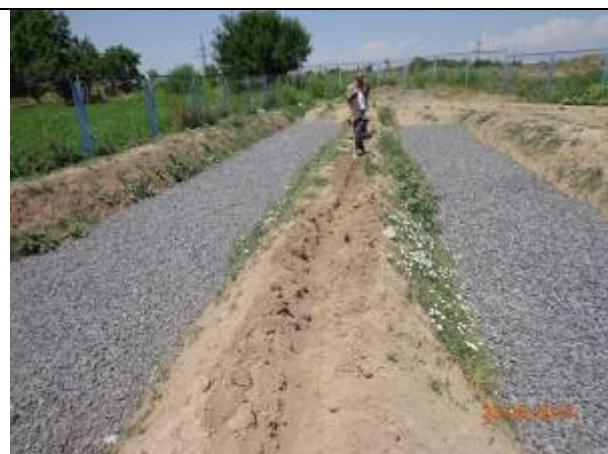
Construction of the sludge bank
