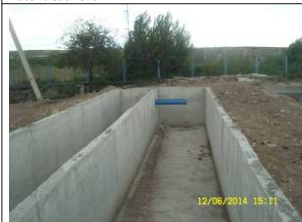
The ferroconcrete sedimentation pool
