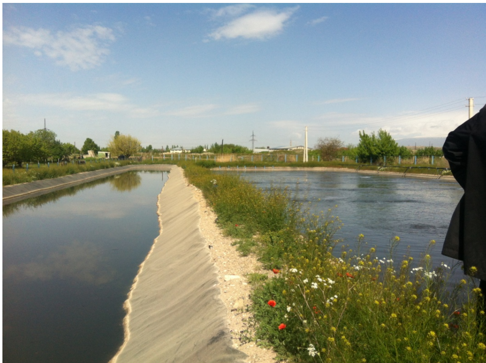
The lagoon systems for domestic wastewater treatment in the Parakar village
