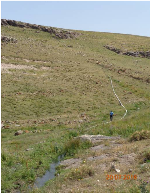
The water pipe-line in the torrent coomb
