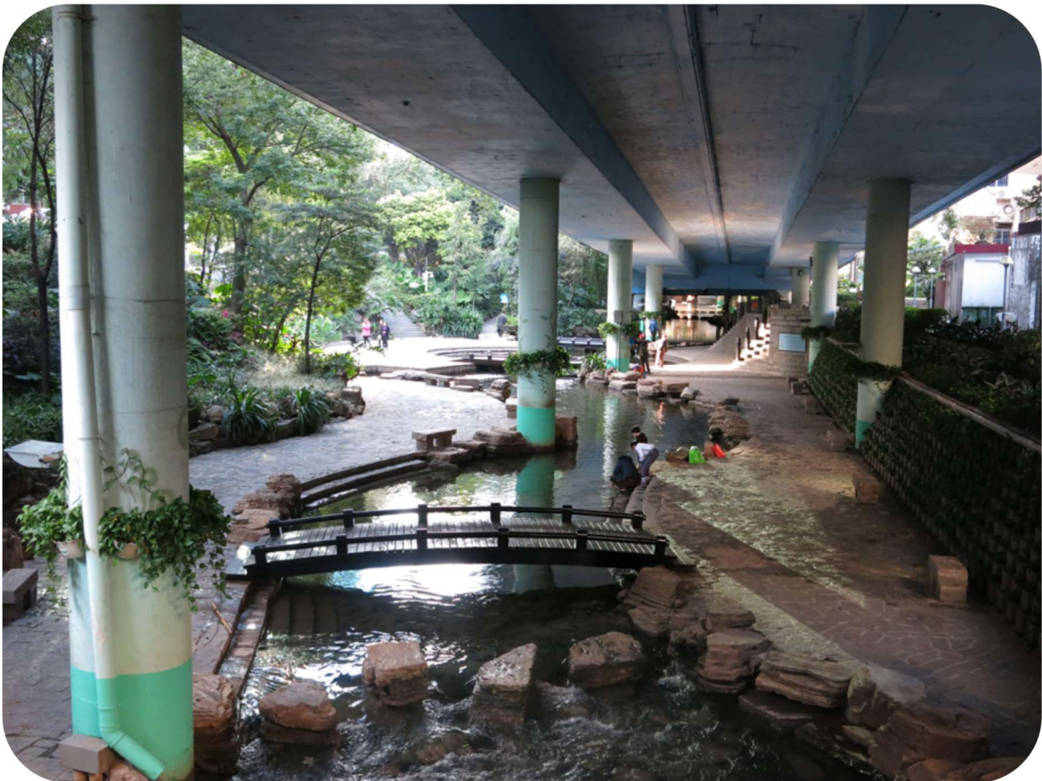
Photo 8: Visit of Guangzhou, Urban River Restoration project, 17 December 2015
