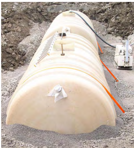
Figure 19. This picture shows the urine tanks at Kullön during the construction process. The tanks will be covered with soil. Photo: Mats Johansson.
