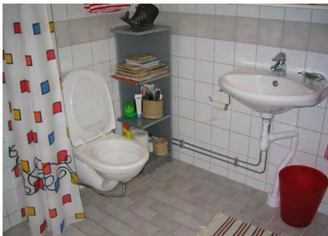
Figure 5. Urine-diverting toilet system at Kullön, Sweden. Photo: Ron Sawyer.
