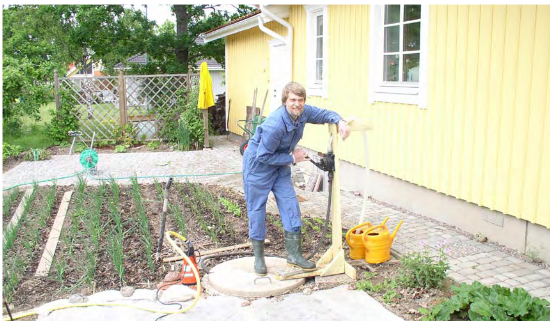
Figure 20. Hand pumping of urine from household tank for subsequent use in garden. Photo: Mats Johansson.
