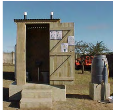
Double-vault urine-diverting toilet with hand washing facility nearby. Photo: Teddy Gounden.
