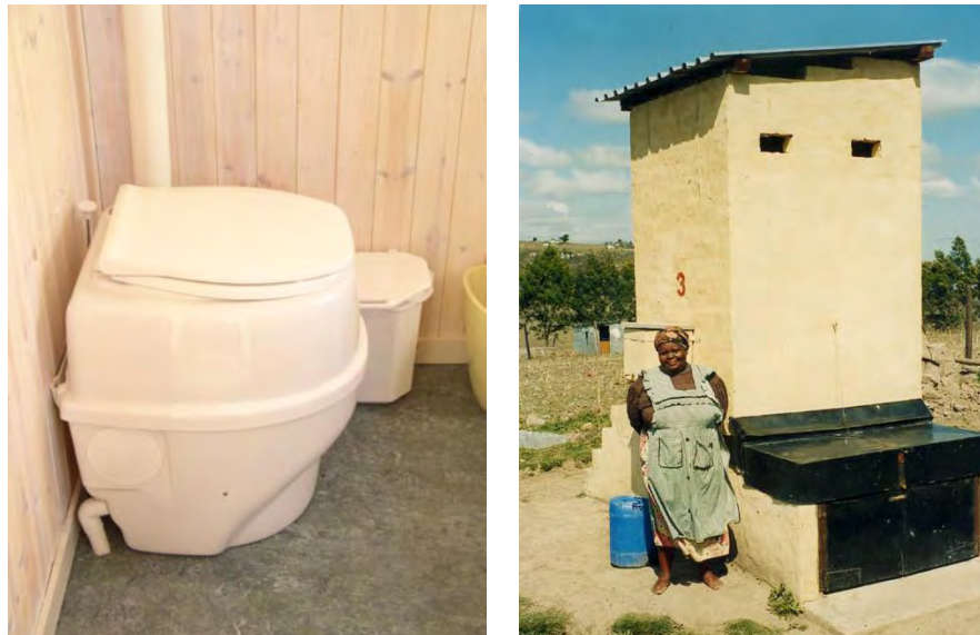
Figure 2. Urine diversion in the on-site low population density context. a) South Africa, photo: Aussie Austin b). Sweden, Separett is a dry urine diverting toilet for indoor use. Photo: Mats Johansson.
