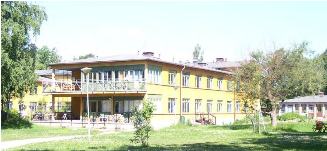
Figure 13. Gebers, once a convalescent home, is today a modern apartment house close to lake Drevviken. Photo: Mats Johansson.
