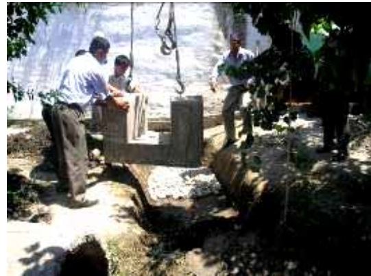
b) Assembling pre-cast flumes
