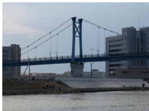
Ural River embankment works in city of Atyrau
