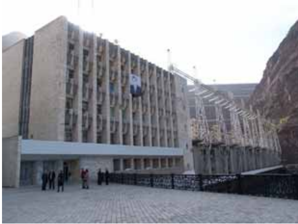
Nurek Hydropower station on the Vakhsh river in Tajikistan
