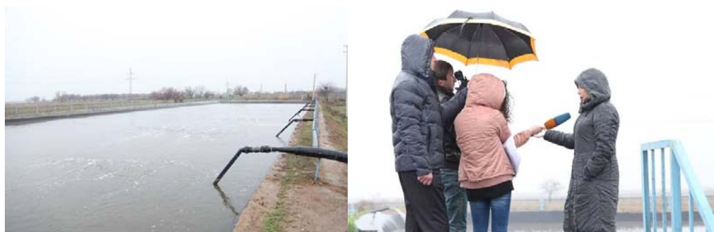
Parakar treatment plant
