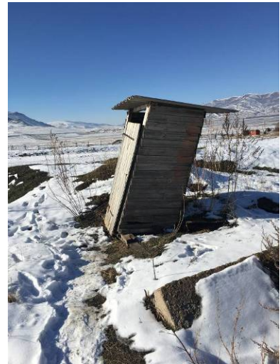
Toilet in the rural school for the upper schoolgirls
