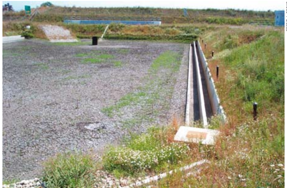
Rainfall water treatment plant in Hoce
