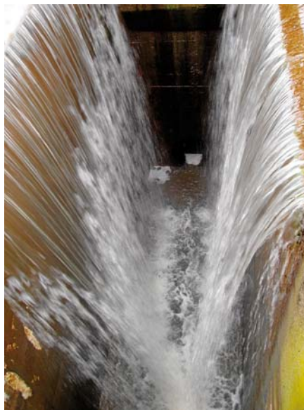
Jelenec Water Reservoir, Slovakia
