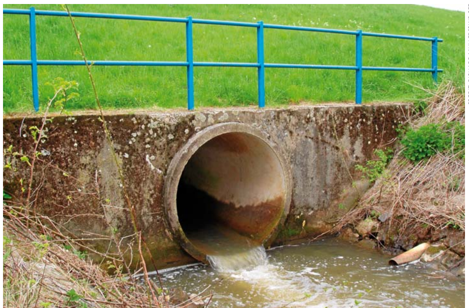
Jelenec Reservoir Water Discharge, Slovakia
