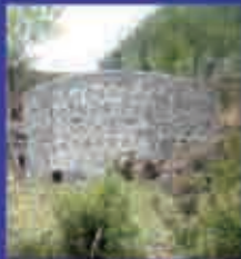
Anti-drought emergency water source project in mountainous area of Daxinhe
