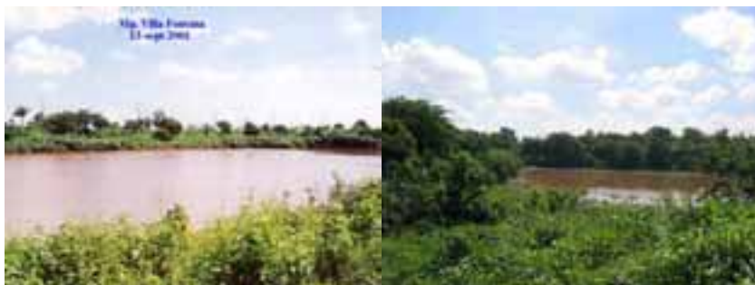
Figure 6.62. Villa Fontana micro-dam in the city of Managua (Source: ALMA, 2005)
