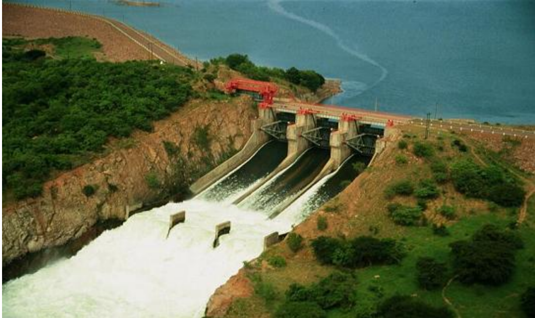
Plate 6: Itezhi-tezhi Dam main spillway (Zesco, 2006)
