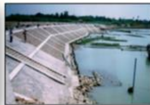
River bank protection works by DWIR
