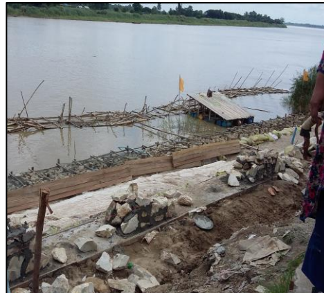
Explanation on River bank protection works of Nyaung don town by U Sein Lwin, Deputy Director, DWIR
