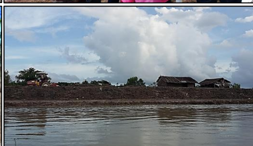
Field visit of Auk Ka Bar sluice gate, Kyat Pha Hmwe Zaung Polder in Pyapon District, operate and maintain by IWUMD
