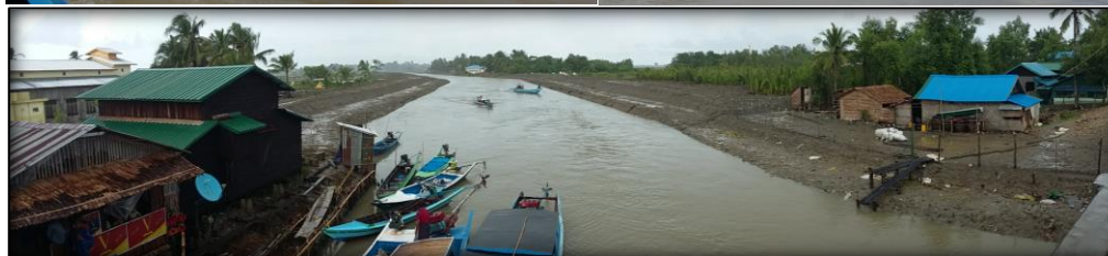
Natural stream re-excavation near Kyet Pha Mye Zaung polder, Pyapon District, Ayeyarwady Region
