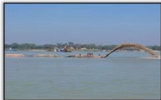
River dredging works
