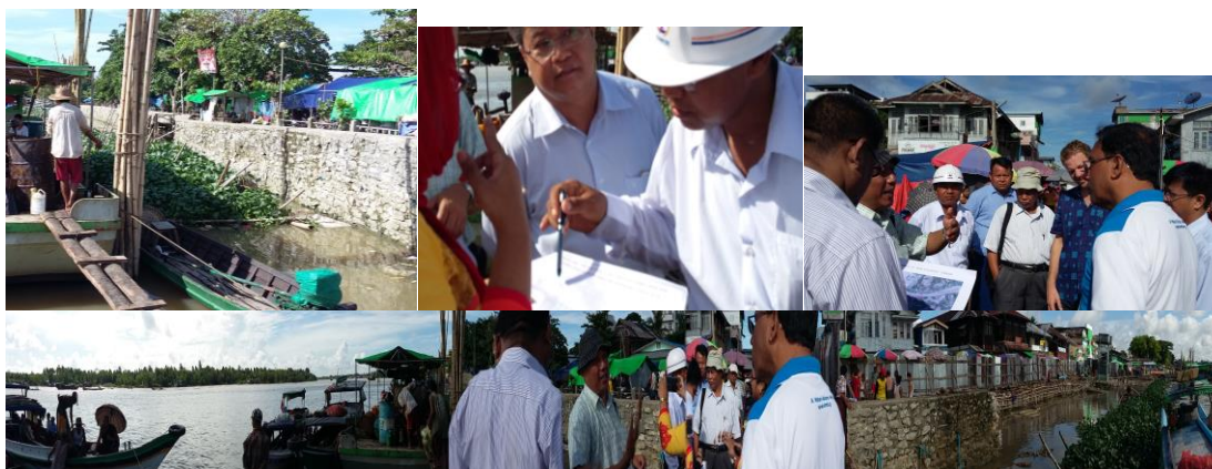
Pyapon town River bank protection works by DWIR
