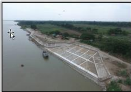
River banks protection works
