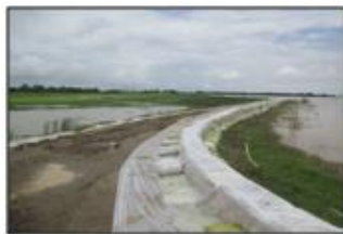
Flood protection embankments by IWUMD (ID)
