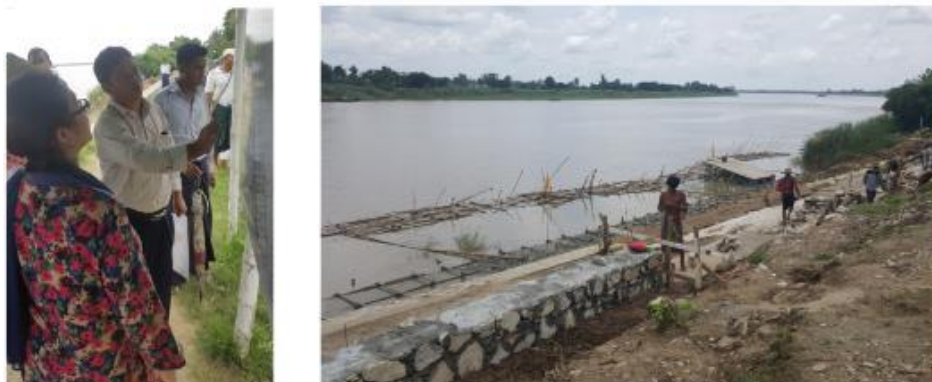
Field trip at Nyaung Done Town river bank protection works
