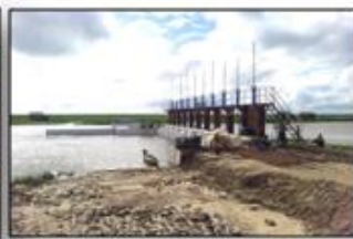
Sluice Gates by IWUMD(ID)
