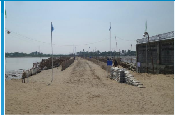
PanHlaing River, Temporary Dyke at RD 174+750
