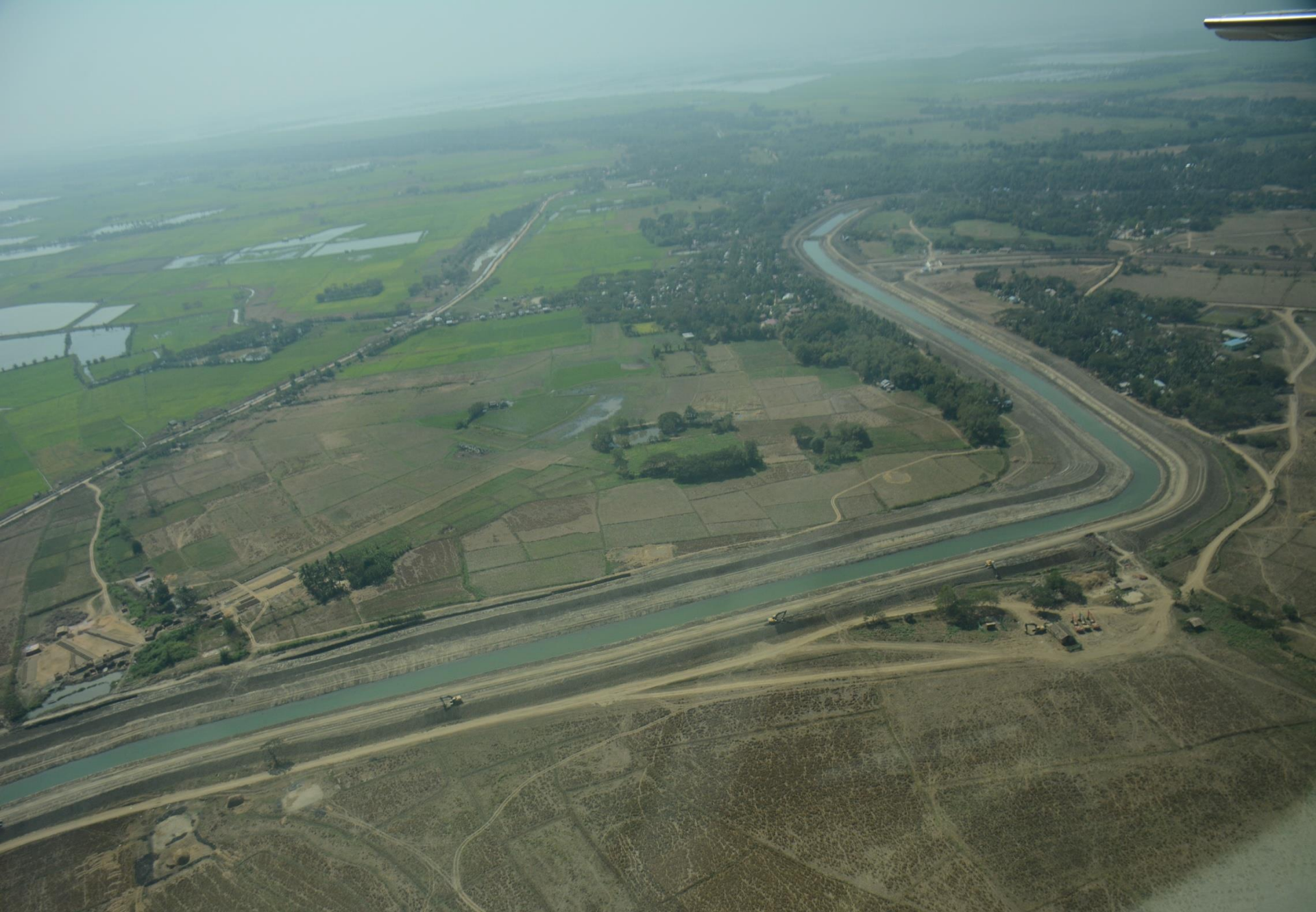
PanHlaing River Rehabilitation Work at RD 46+000 to RD 50+000
