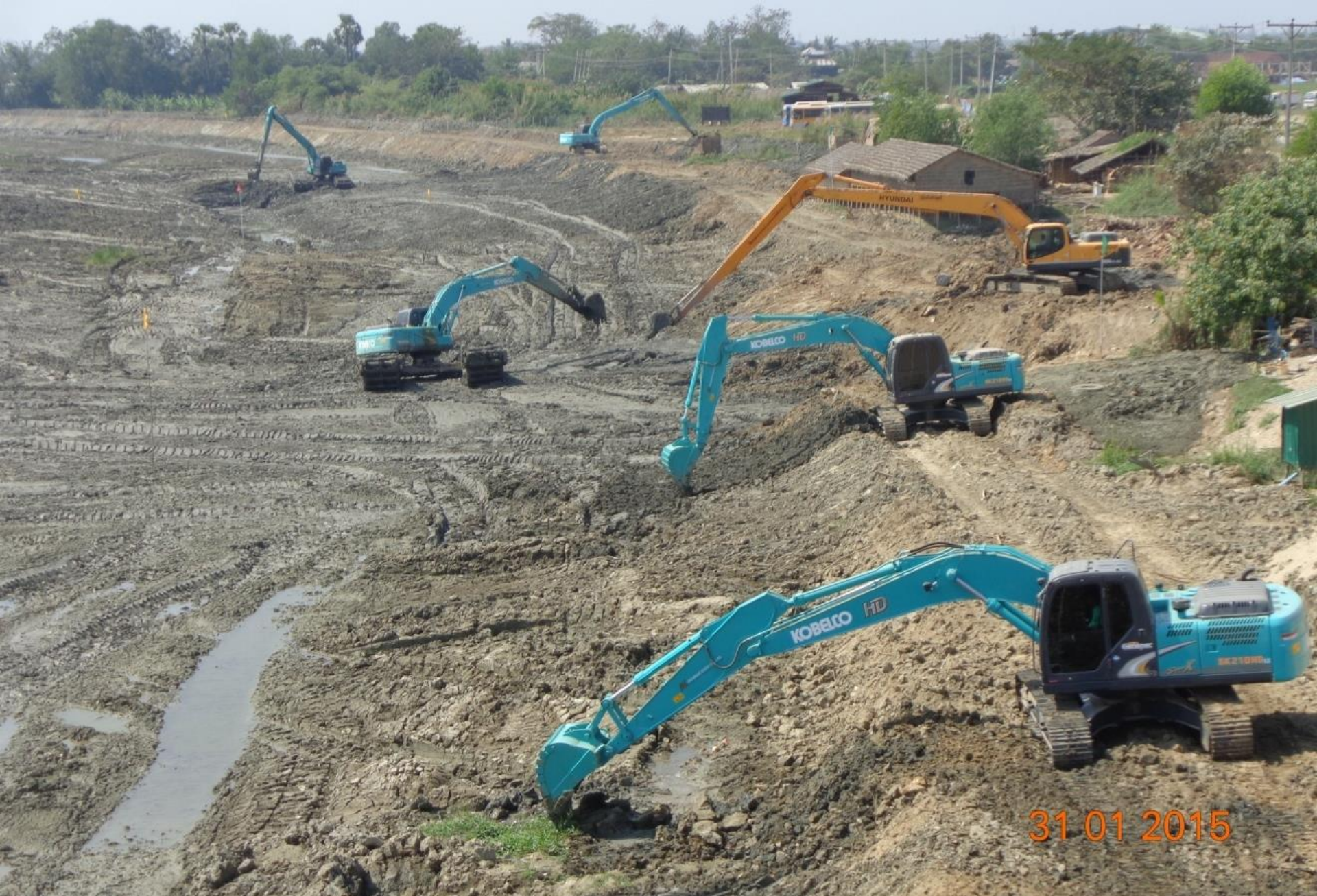
PanHlaing River Rehabilitation Work at RD 145+000
