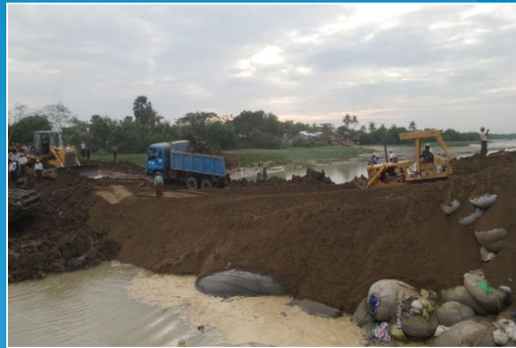
PanHlaing River, Temporary Dyke at RD 174+750
