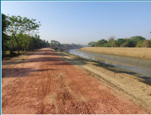
RD 8+000 to RD 10+000 Embankment / Gangar Road way
