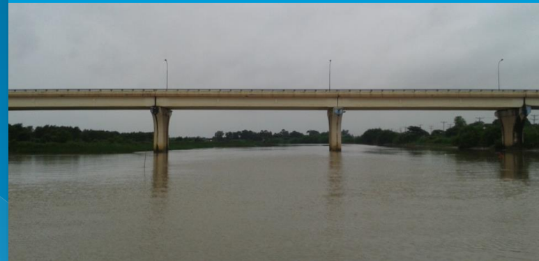
Highway bridge crossing PanHlaing River (R.D-150+600')
