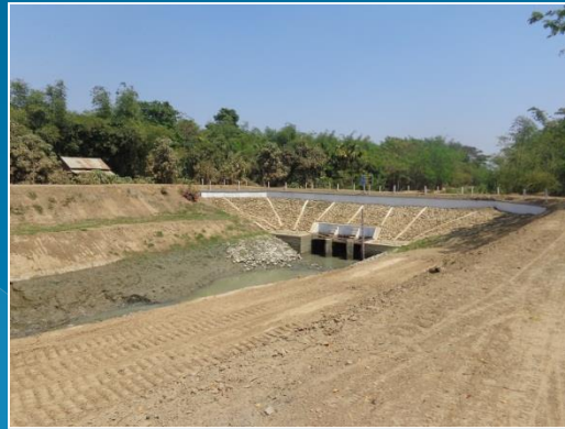
RD 10+000 Than payar creek sluice
