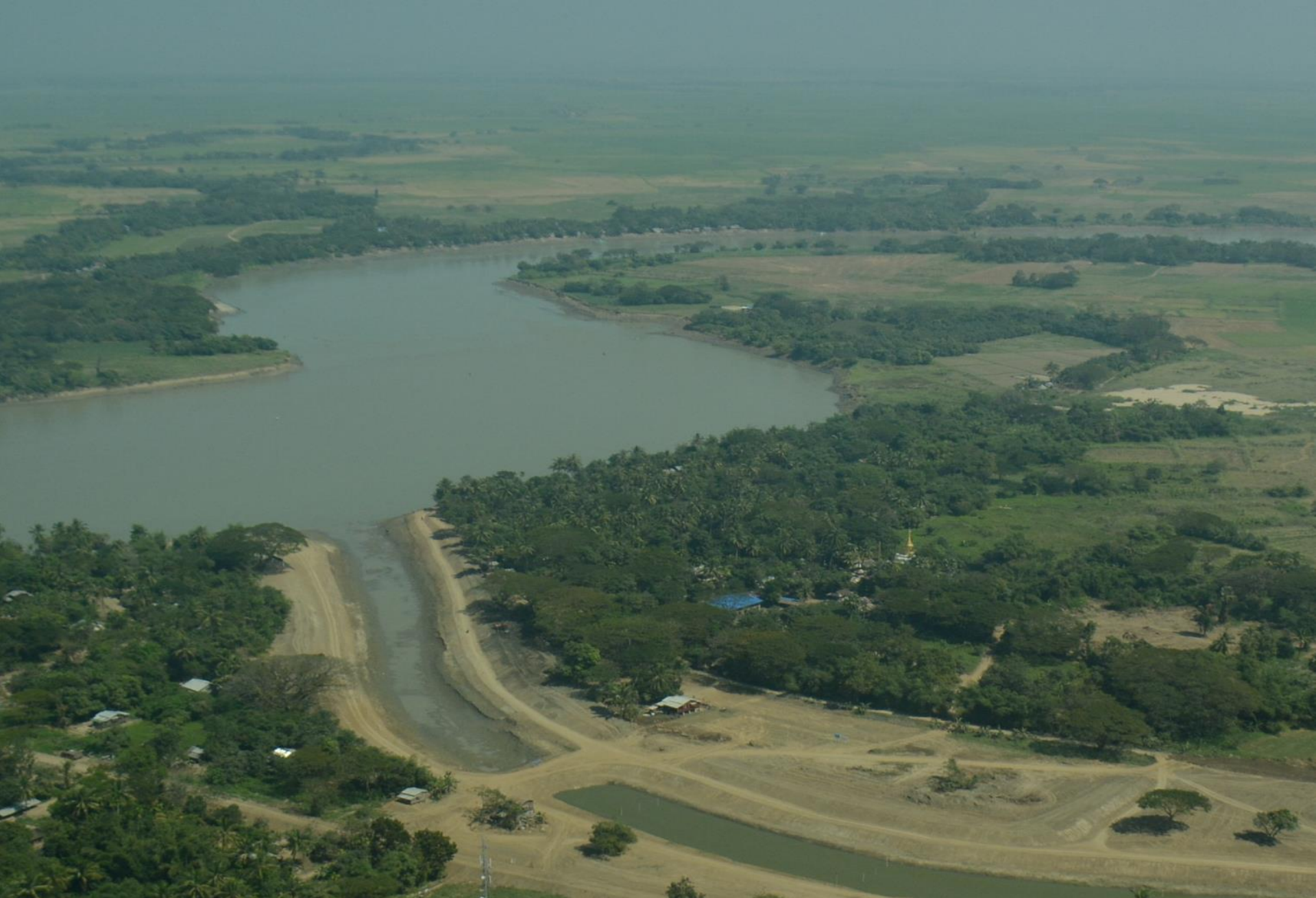
PanHlaing River Rehabilitation Work at Confluence of Kokkowa River and PanHlaing River (RD 0+000)
