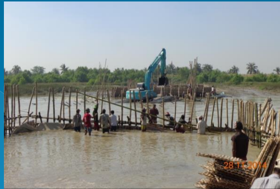
PanHlaing River, Temporary Dyke at RD 158+000
