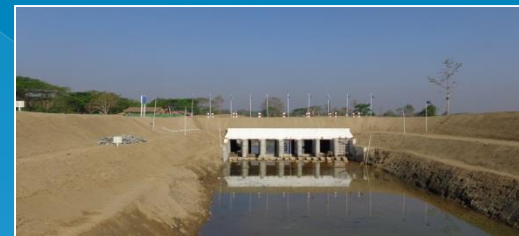
Mya Ge sluice gate, RD 46+000
