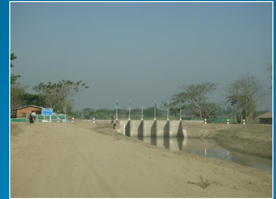
RD 56+000 Mingalar sluice gate
