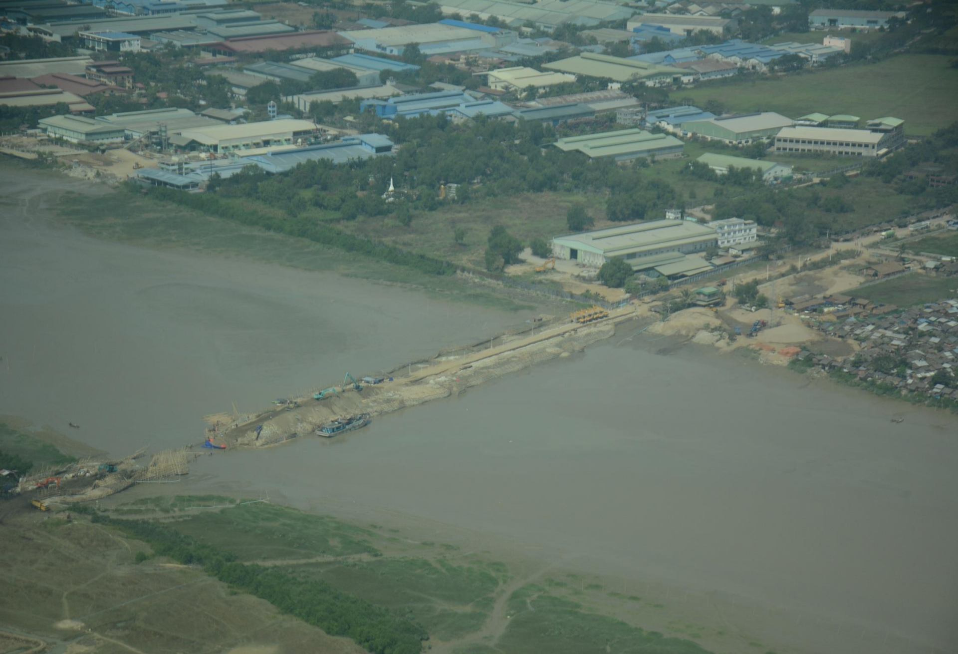
Temporary Dyke Construction at RD 175+000
