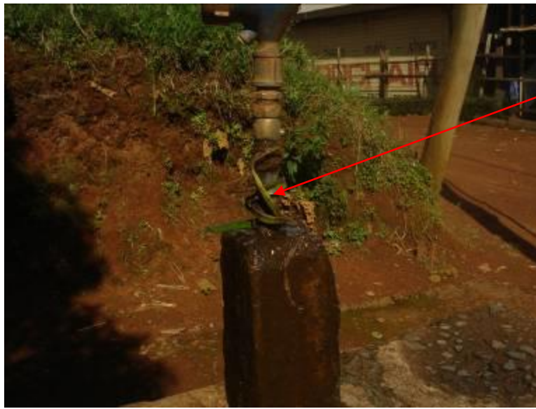
Figure 2: Poor craftsmanship for leak repair at a public standpipe
