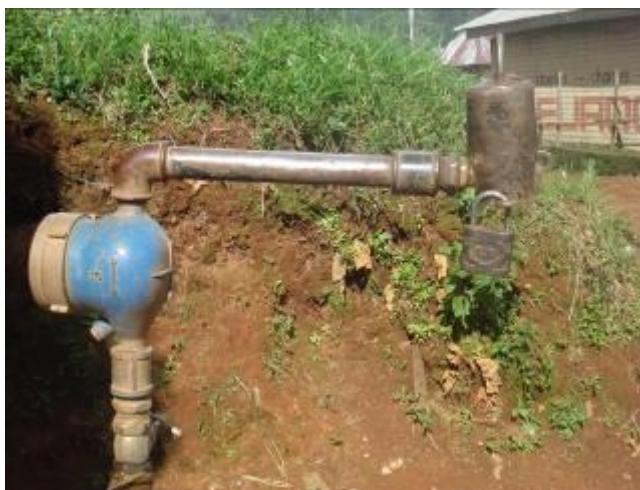
Figure 1: Public standpipe with meter and lock (picture by author in the afternoon- period of low demand)
