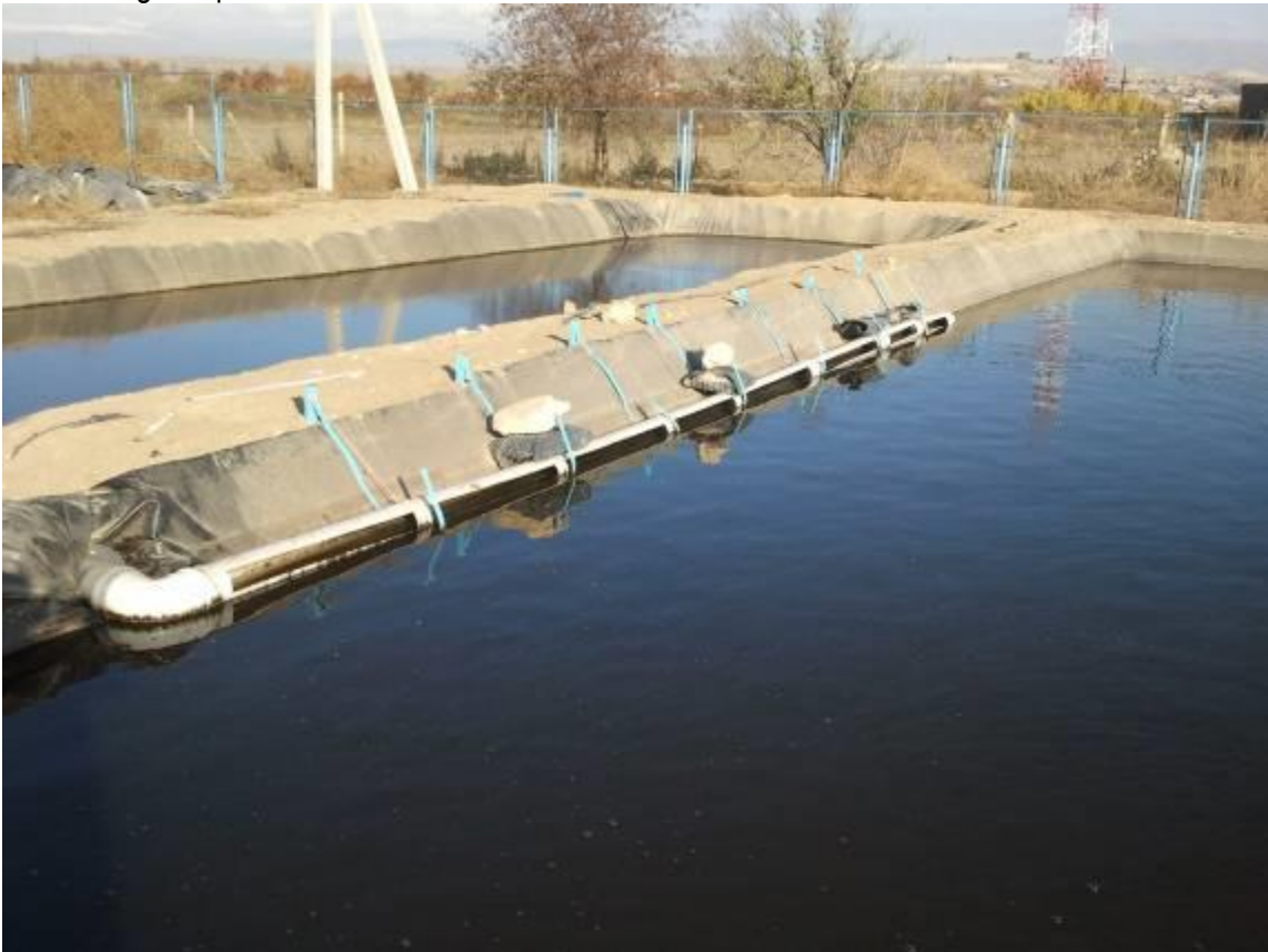
Figure 2. Details of the lagoon type of wastewater treatment system in Parakar village
