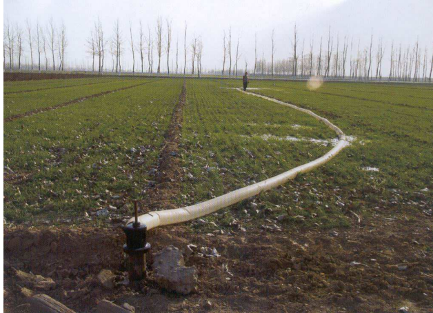
Figure 1. Pipe Water Supply and Border Irrigation Site
