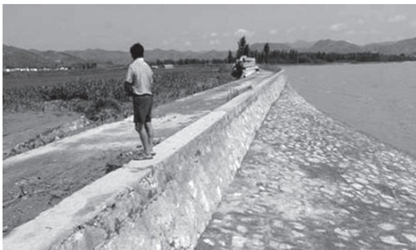
Dike protection, Hubei Province, August 2007
