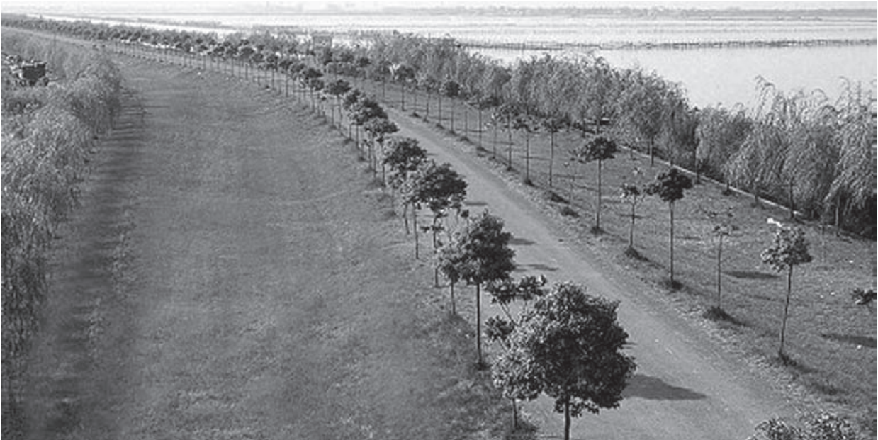
Flood control dikes, Yellow River
