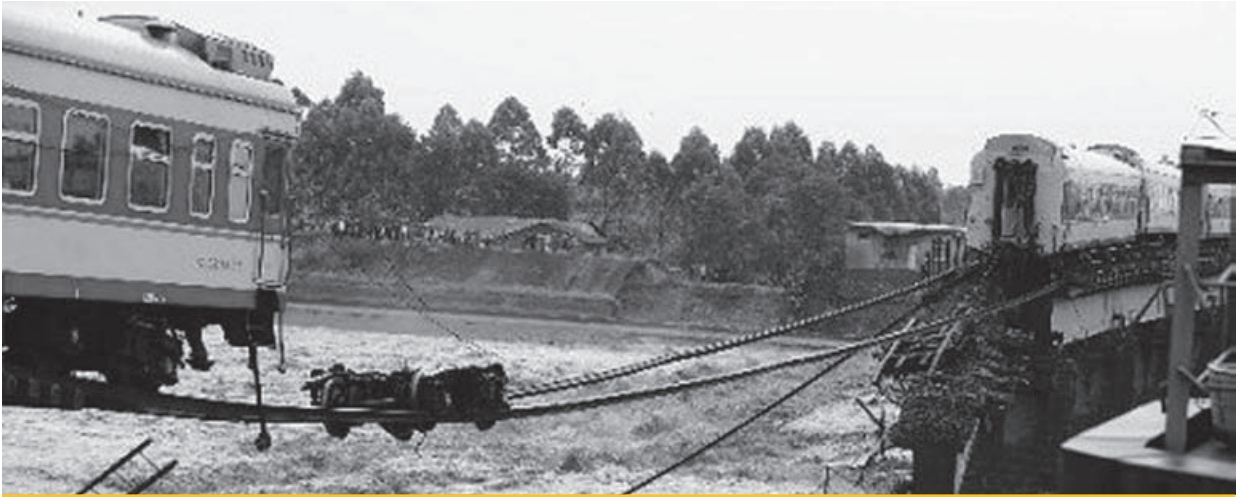
Rail bridge collapse
