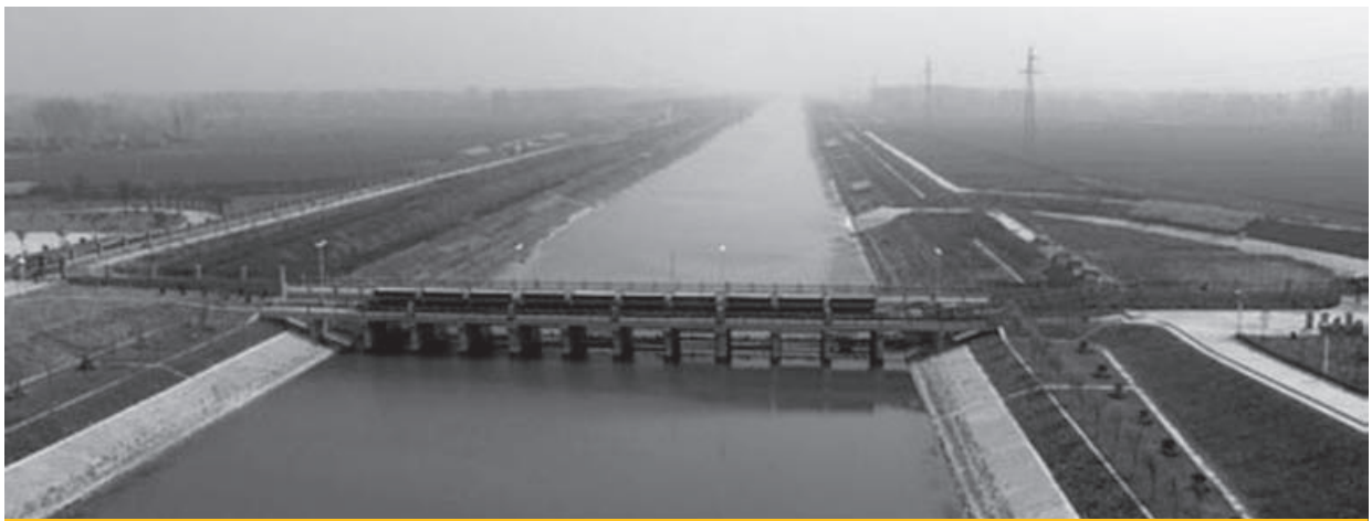
Flood diversion channel
