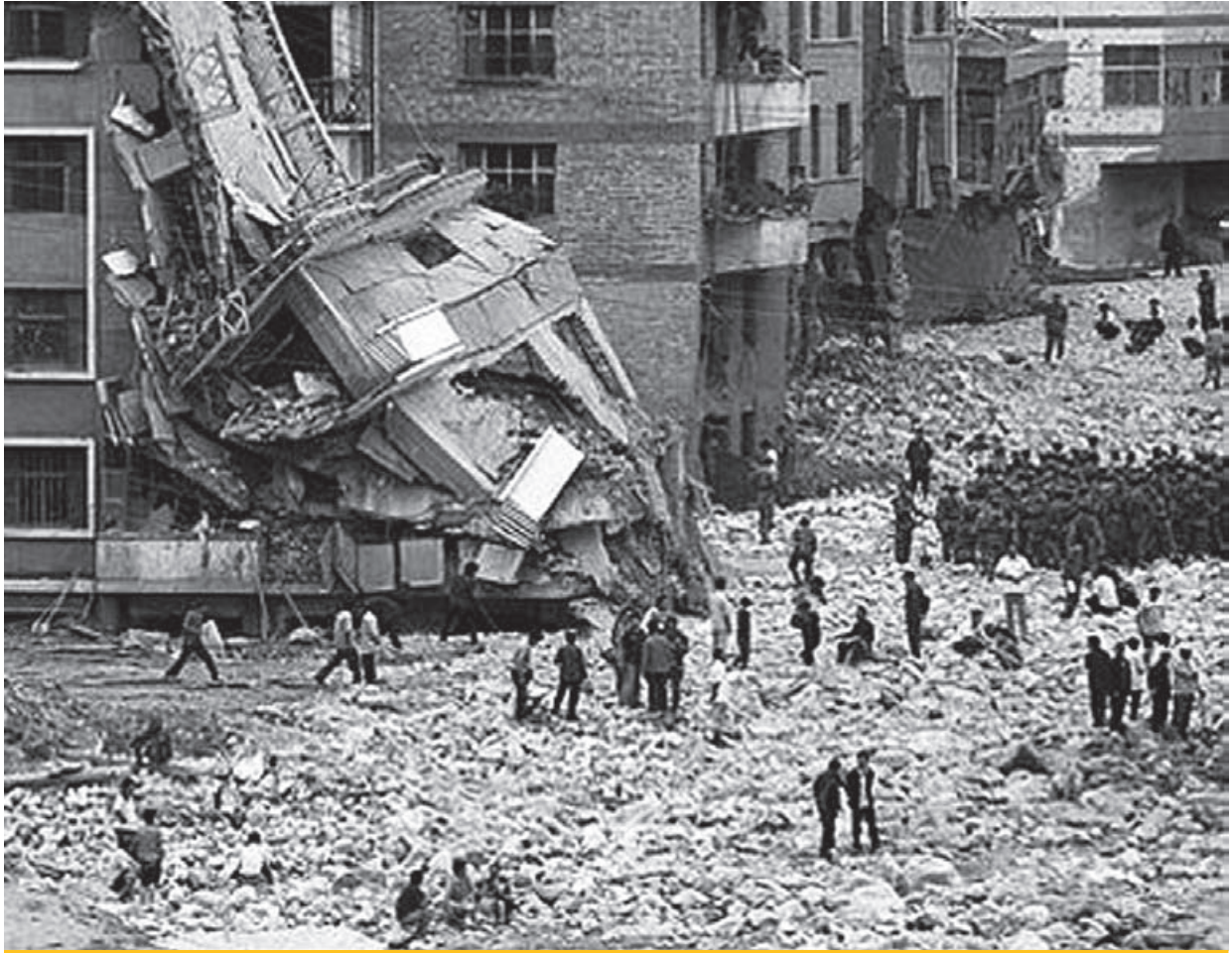
Damages after the debris flow, Zhouqu County, Gansu Province, September 2010
