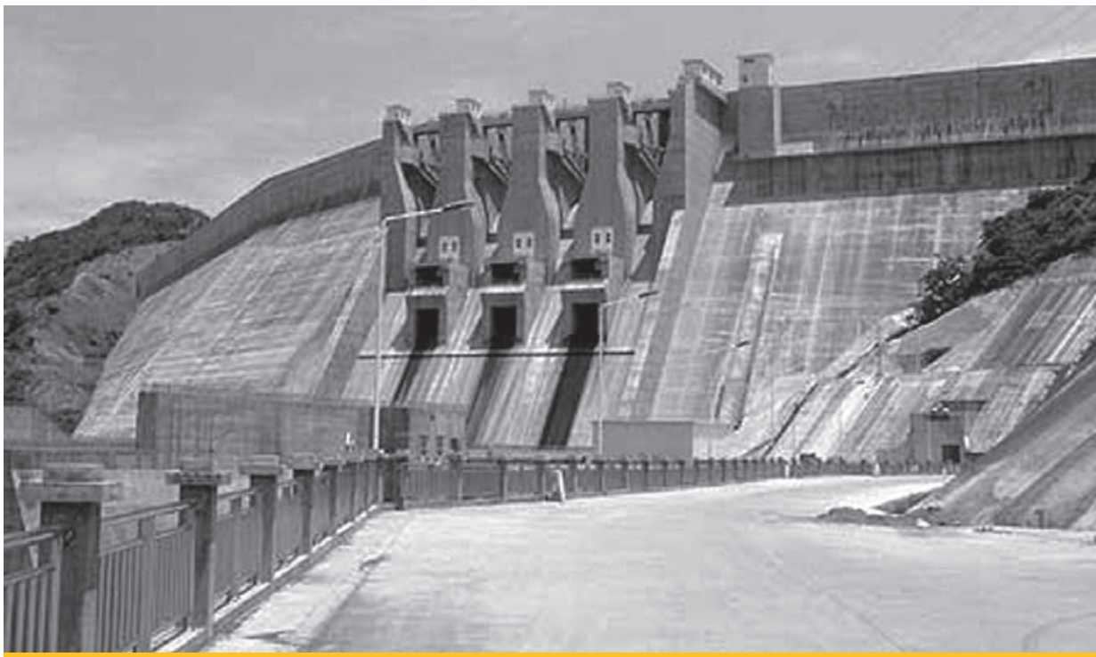
Flood control reservoir, Baise County, Guangxi Zhuang Autonomous Region
