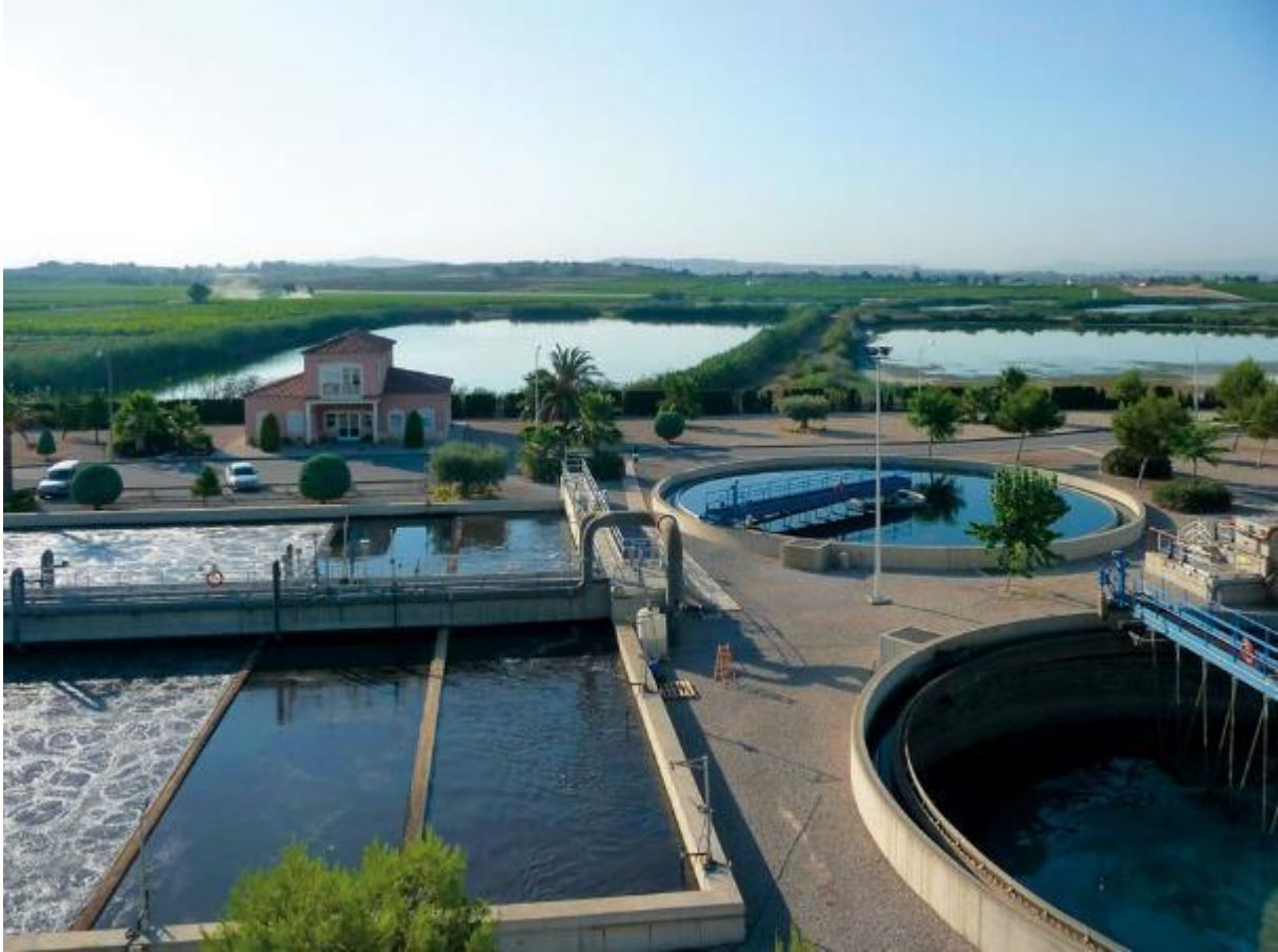
Figure 3: Waste Water Treatment Plant of Mazarrón
