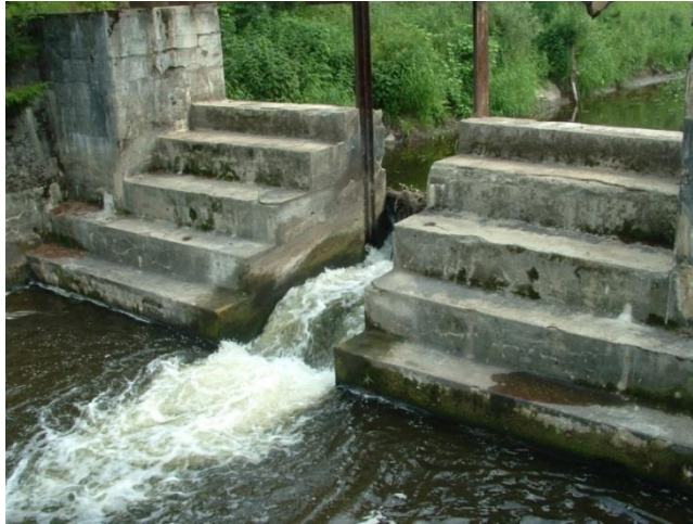
Photo 1. Damming device on the channel constructed in the 1920s
