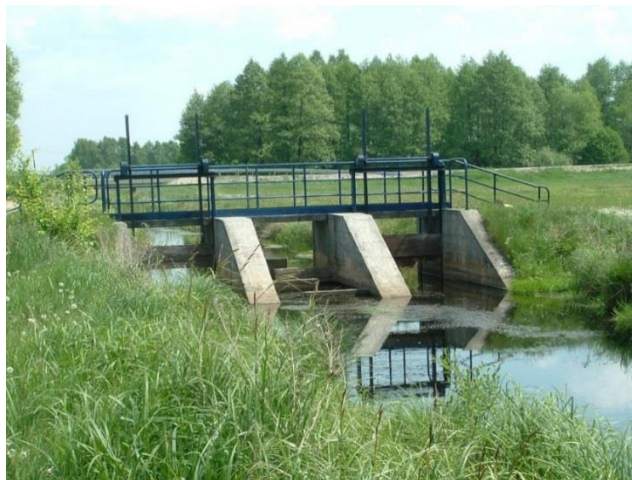
Photo 6. Hydraulic structure in the Kampinoski National Park – wetlands protection
