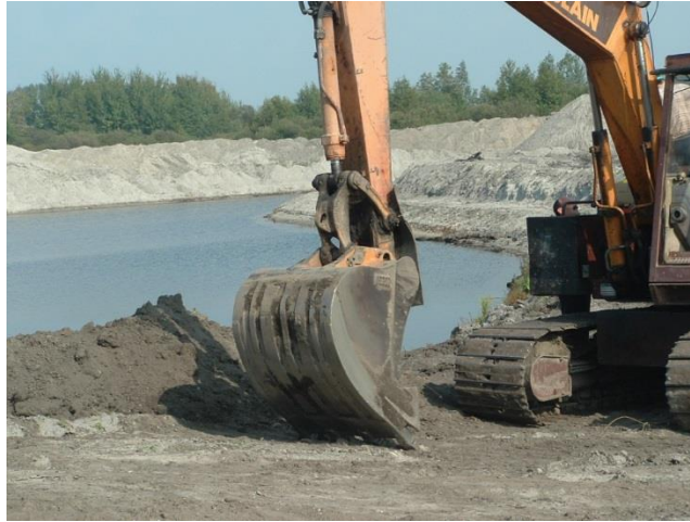
Photo 7. Construction of the reservoir in the river valley
