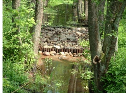
Photo 5. Stone threshold – small retention in forests
