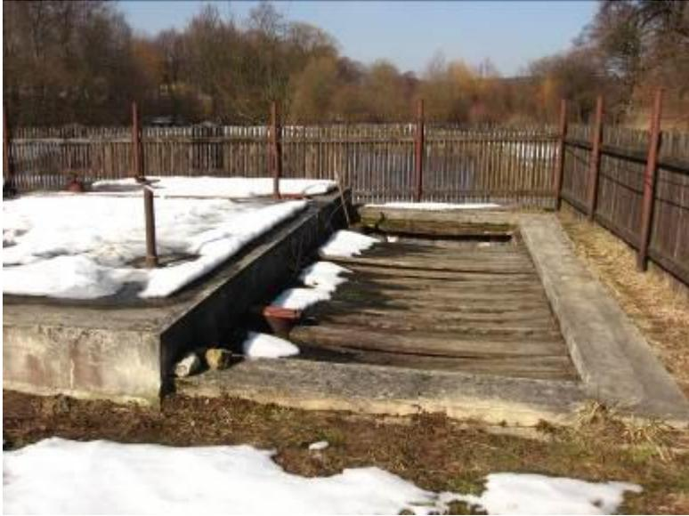
Shallow combined settling tank with a lateral sludge digestion compartment
