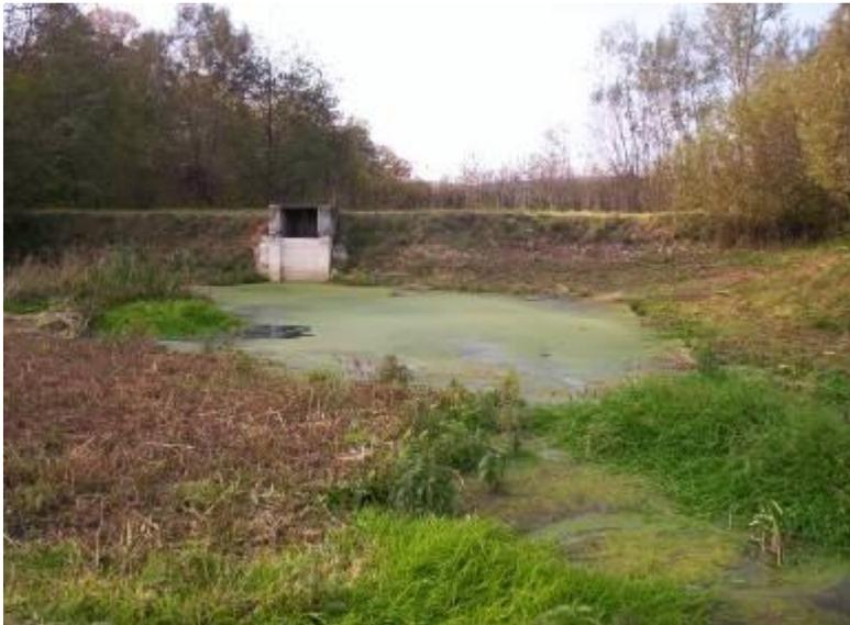
Outflow structure – simple half-closed gullet with a simple sluice plank wall
