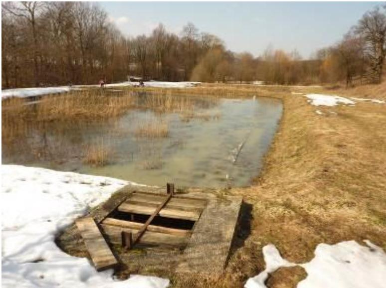
Elevating of the water surface level within the constructed wetland filter in a spring time
