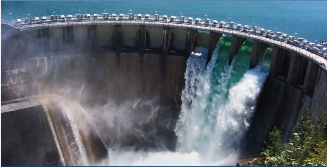
Kerr Dam on the Flathead River, USA
