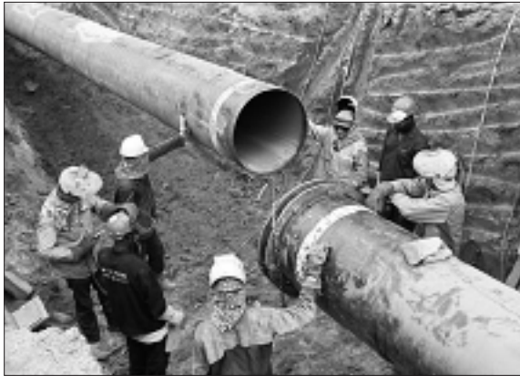
Building the Chad-Cameroon pipeline
