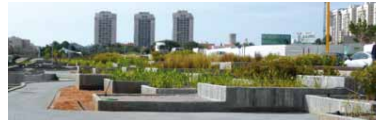
Tel Aviv pocket wetlands using treated grey-water from neighboring apartment buildings.
