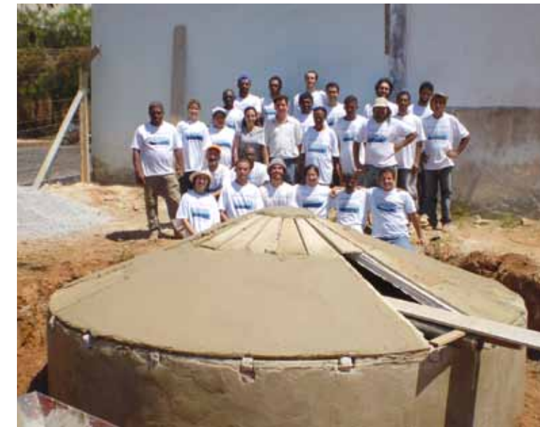
BH Stormwater Collector at Barreiro Productive Garden (Thiago Salles).
