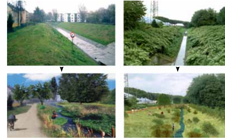
Naturalising stormwater channels in the Emscher Region.
