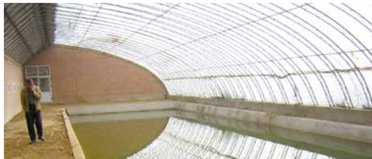
Huairou Cooperative Greenhouse Rainwater Harvesting System.
