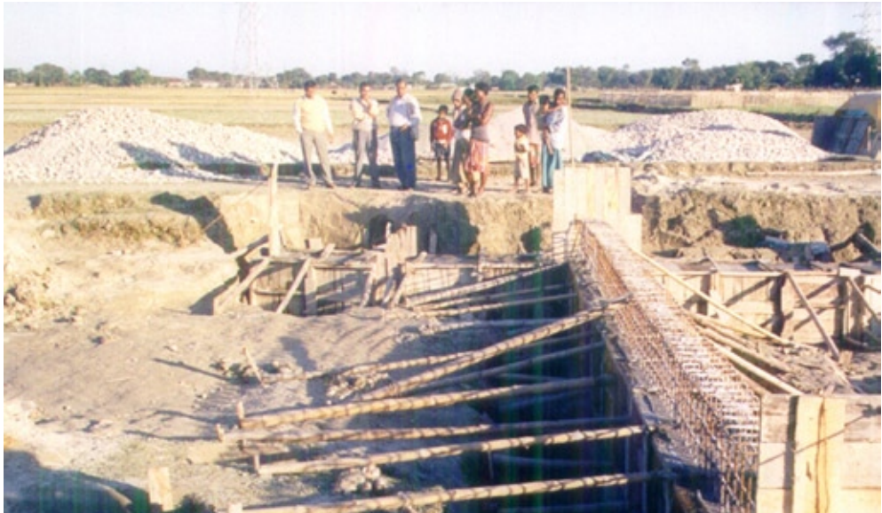
Figure 2: Constructing a gully plug to retain groundwater
