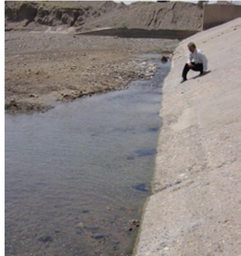
Figure 3: Water emerging from weepholes
