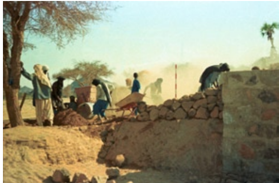
Figure 2: Construction of diversion works
