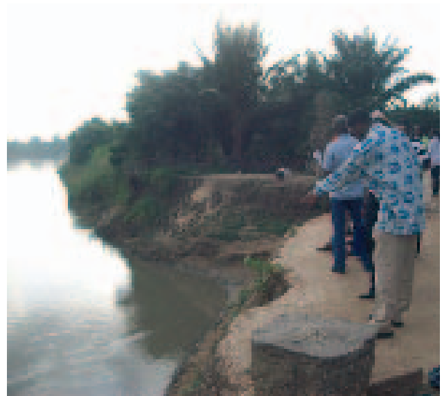
Erosion of the river bank in Athieme
