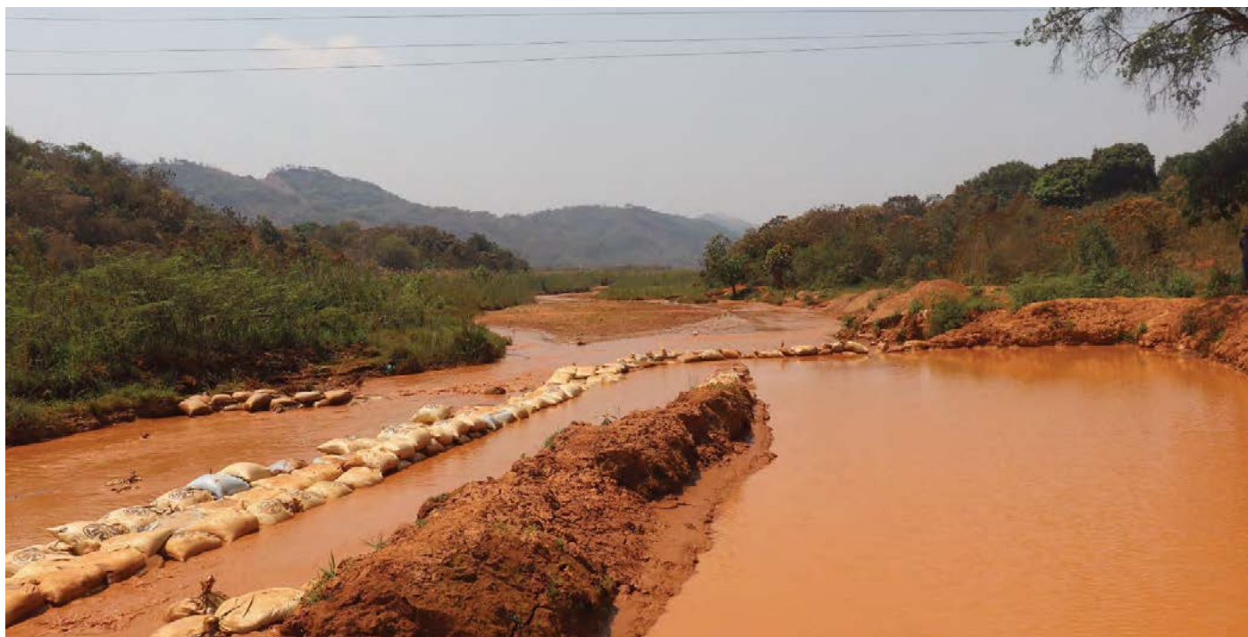
Makeshift tailing dams made by artisanal miners in Penhalonga, Mozambique, in an attempt to address the compromising quality of water due to unsustainable mining practices in the tri-basin. Photo credit: Davison Saruchera
