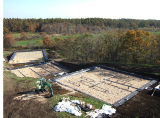
A combination of two vertical subsurface flow wetlands and a Horizontal subsurface flow wetland
