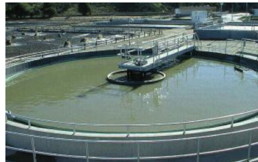
Circular primary sedimentation tank
