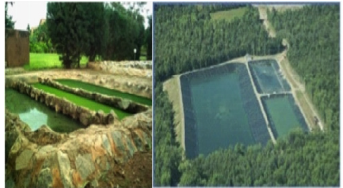
Mini Waste Stabilization Ponds consisting of a anaerobic (right), facultative (middle) and aerobic pond (left)
