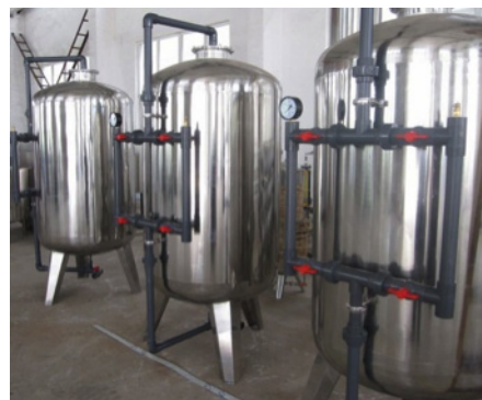
Activated carbon filtration units for groundwater treatment
