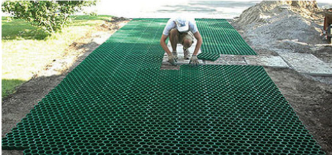
Pervious pavement in a parking lot
