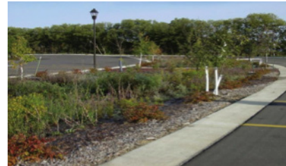
Bioretention Cell in Parking
