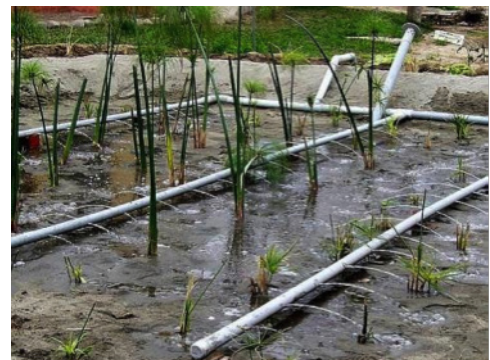
Vertical subsurface flow wetland
