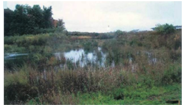
Free-surface flow type constructed wetland
