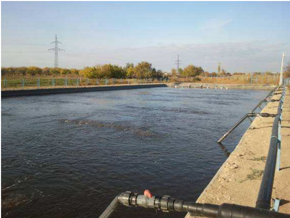
Figure 1. Lagoon type of wastewater treatment system in Parakar village
