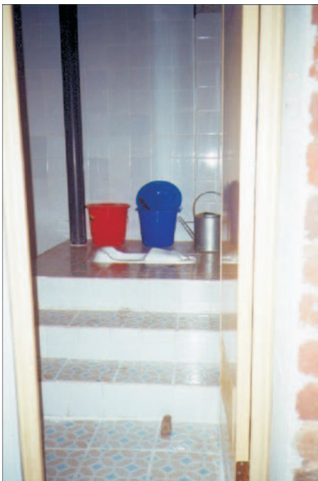
Figure 16. Indoor urine-separating toilet with squatting pan in China
