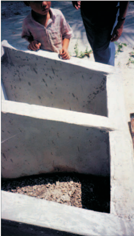
Figure 13. Collection of faecal material should preferably be done in twin pit compartments. When full, one pit is sealed off and the storage time counted from that date, while the other pit is used. In Vietnam, representing a hot climate a full destruction of Ascaris eggs and model viruses were obtained within six months during these conditions. If twin pits are not used, secondary storage or other types of treatment must be planned for.
