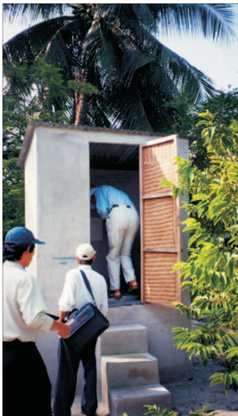
Figure 17. Elevated urine-separating toilet in Vietnam
