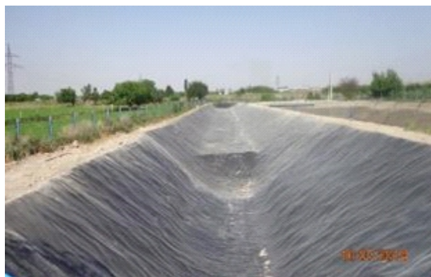
Photo: the second pond for sewage treatment with natural aeration
