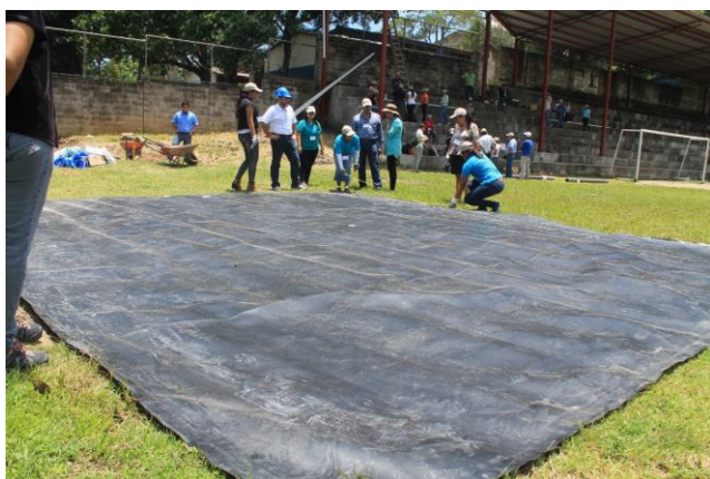
Image 1: Installing the bag in Jerusalén
