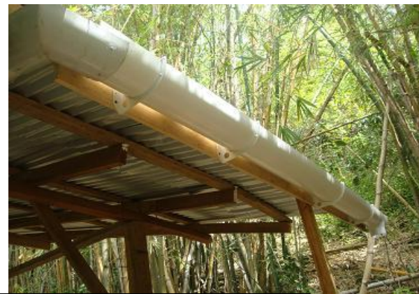
Cross-section of the guttering for the Rainwater Harvesting (RWH)
