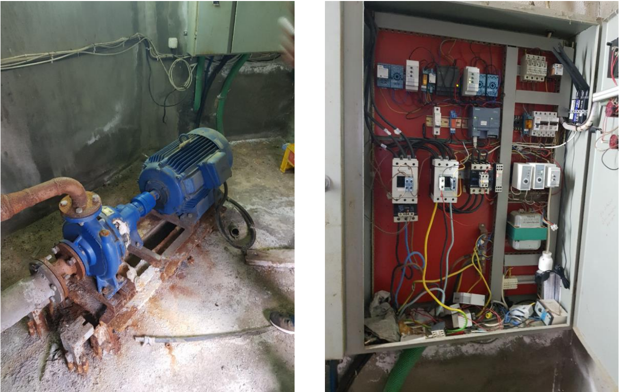
Picture 5. The Aspoxomata pumping station
