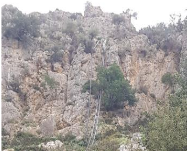
Picture 2. Pipelines to be replaced and supported.
