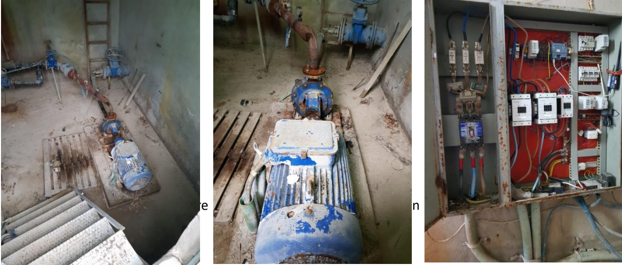
Picture 4. The Mesarmos pumping station
