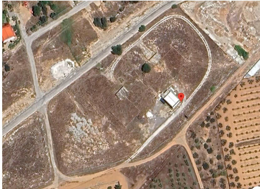
Figure 2. The Water Treatment Plant of Corinth
