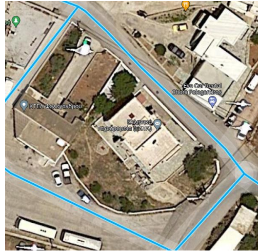
Picture 5. The roof of the municipality building
