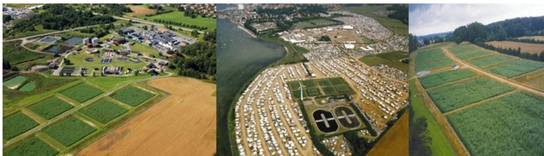
Figure 1: Reed beds in Denmark: Skövde (2003, 1.200 tonnes of dry solids per year; left), Rudkøbing (1992, 250 tonnes of dry solids per year; middle), and Kolding (1998, 2.000 tonnes of dry solids per year; right) 4
