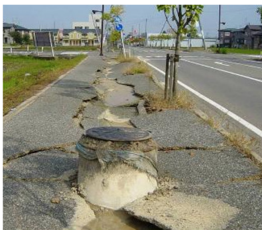
Figure 5: Manhole buoyancy consequences 29 and manhole with double bottom 30 prevents deformation
