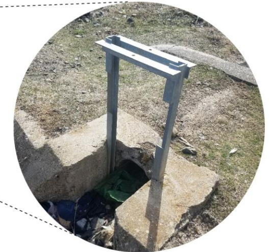
Gate in secondary canal - MISSING
