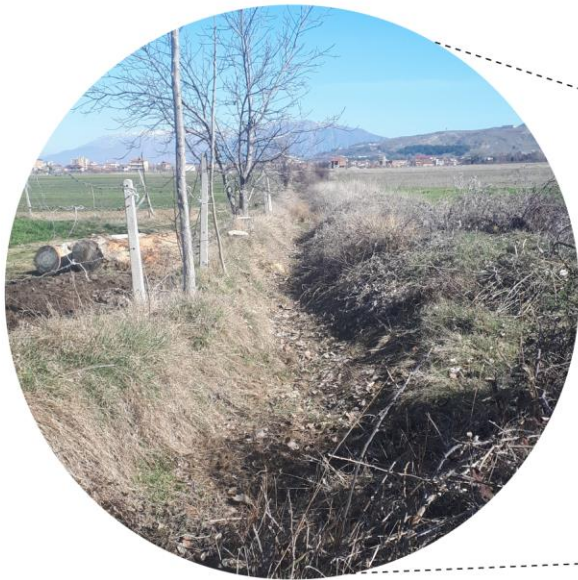
Secondary canal - OUT OF FUNCTION (6.4 km)
