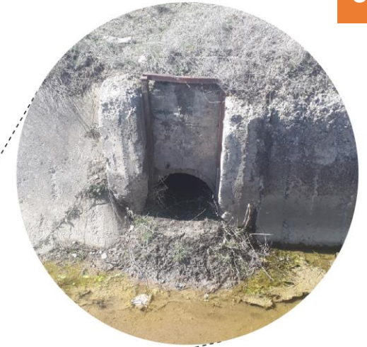
Outlet in primary canal - MISSING
