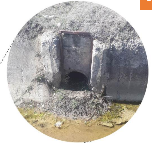
Outlet in primary canal - MISSING
