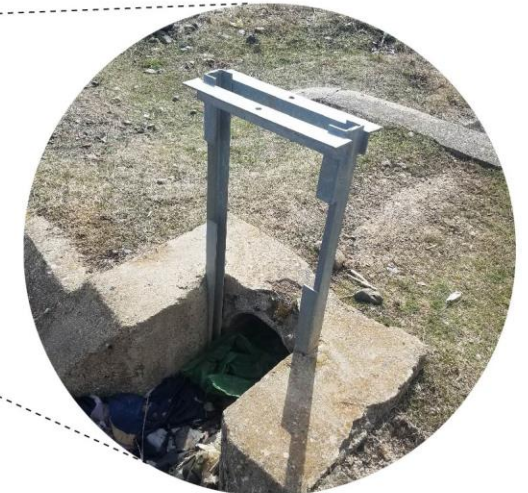
Gate in secondary canal - MISSING
