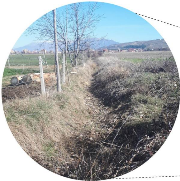
Secondary canal - OUT OF FUNCTION (6.4 km)
