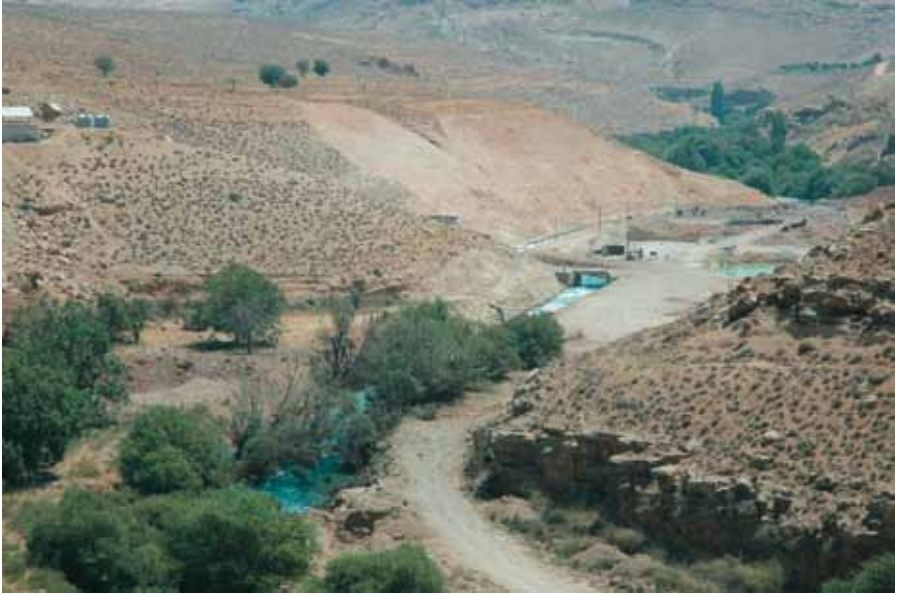
Figure 1: Diversion dam before the bombing © Georges Comair
