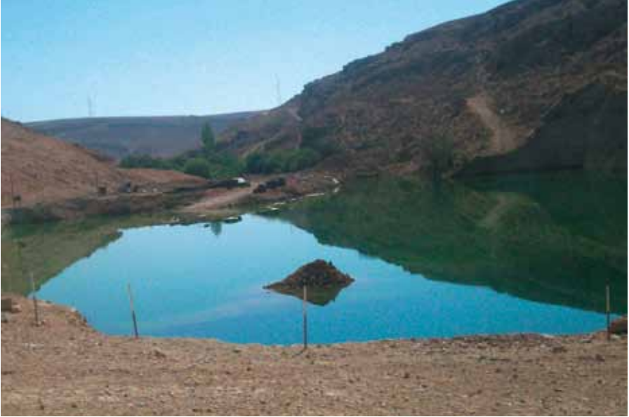
Figure 2: Diversion dam after the bombing © Georges Comair
